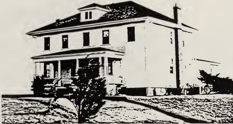
NEED Collaborative - Tract #17-2710 Bldg #T-116
